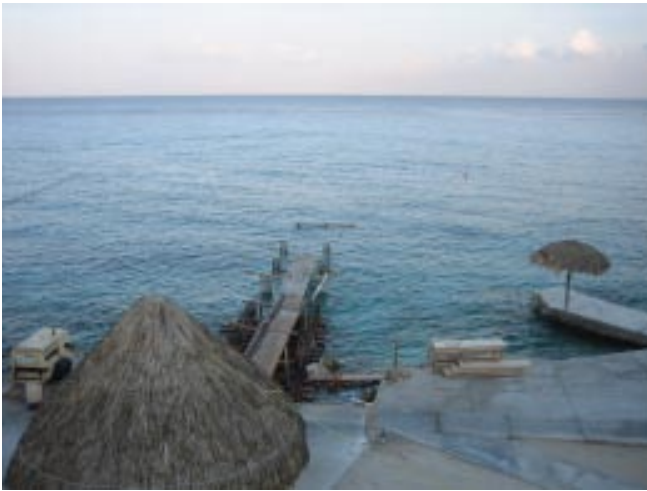
Work on the new dock
